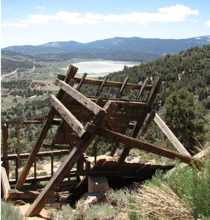
Head frame at the Lucky Baldwin Mine Baldwin Lake in the background (Big Bear summer field trip)
